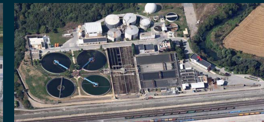
Crisprijana WWTP in Vitoria
